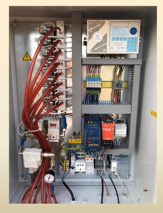
The heart of the control unit is a CPU that control and display the ring functionality and its regulation.
